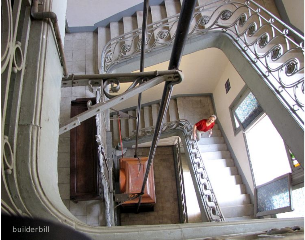
Img 6.3.1: A generous sized stairwell
