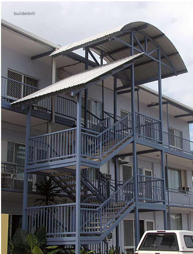
Img 11.2.3: A shaded stair tower
