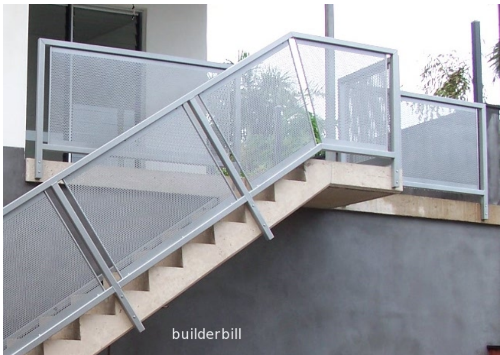
Img 7.0.10: Side fixed balustrades
