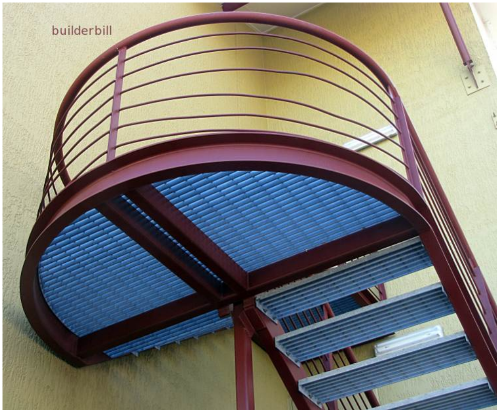
Img 11.1.2: Fire Escape Stair
