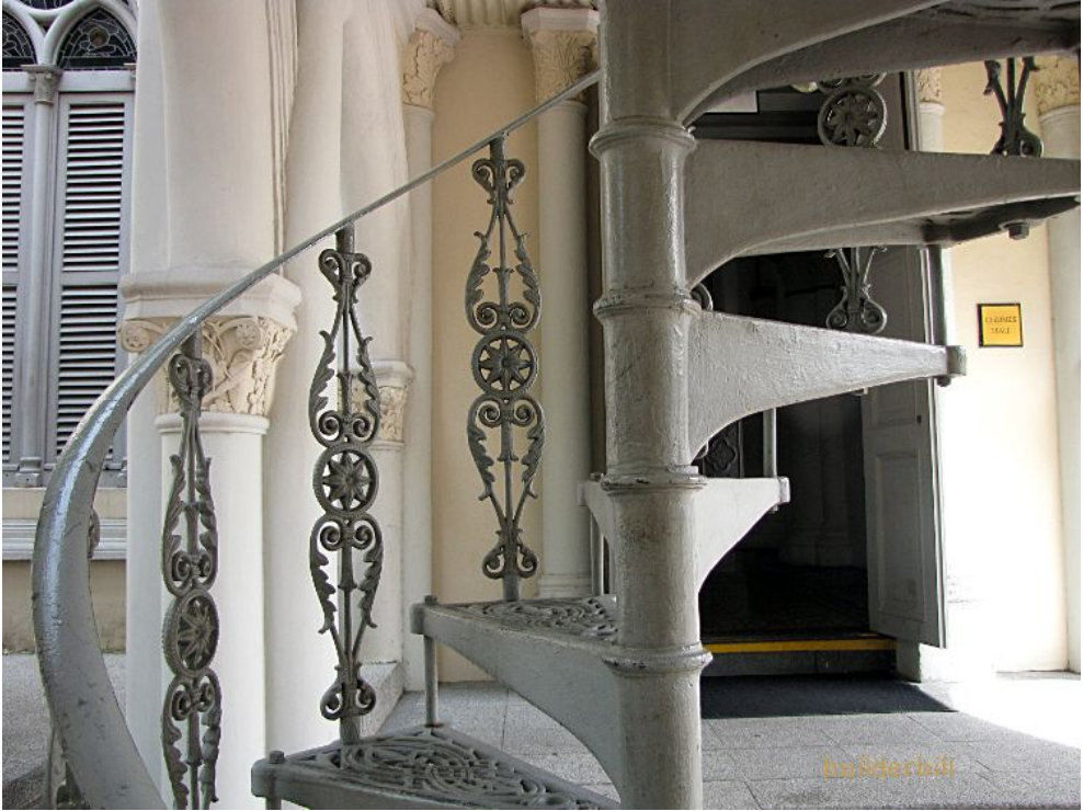
Img 5.4.1: A spiral stair around a central column.
