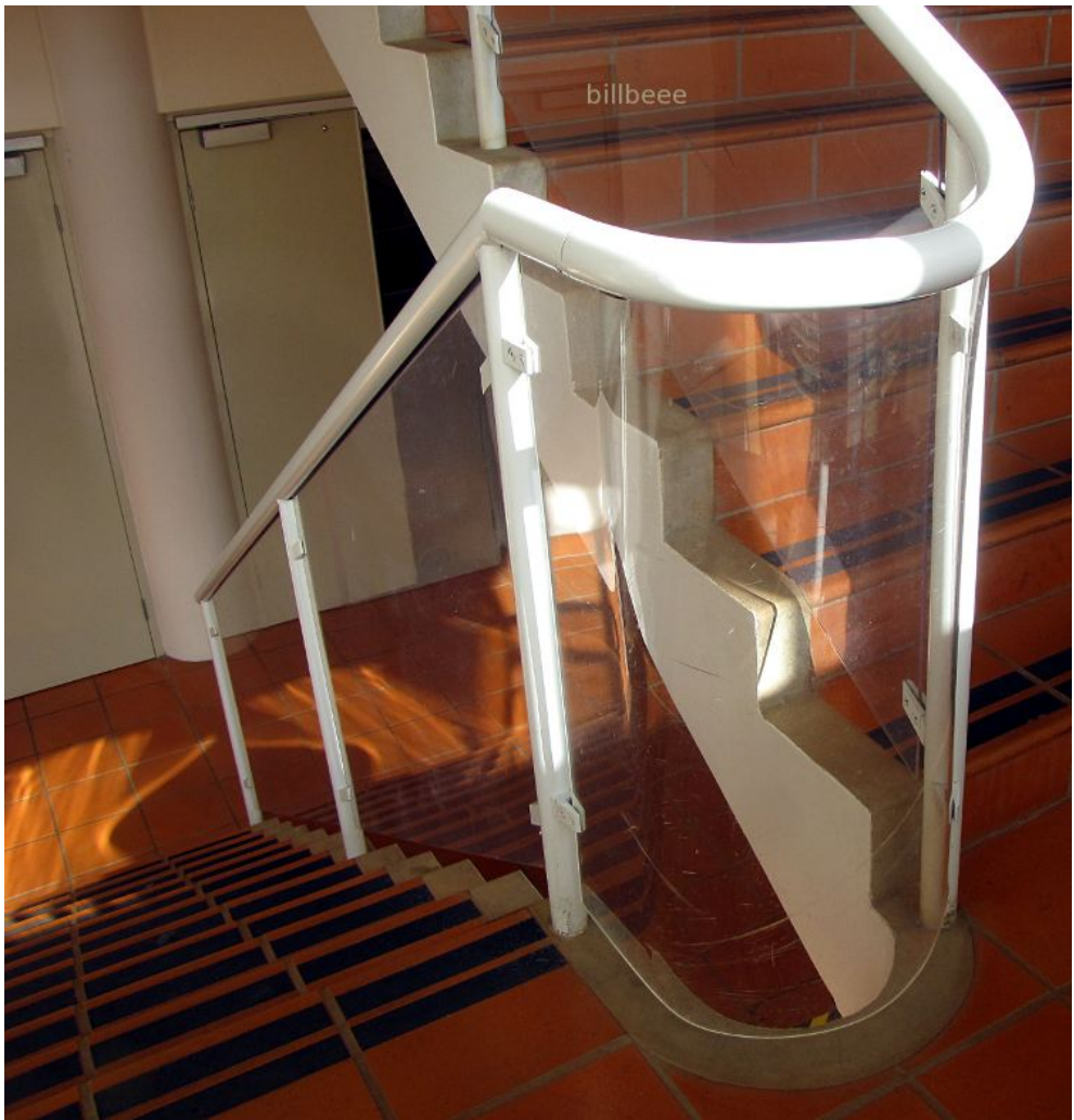
Img 7.0.9: Moulded Perspex Balustrade
