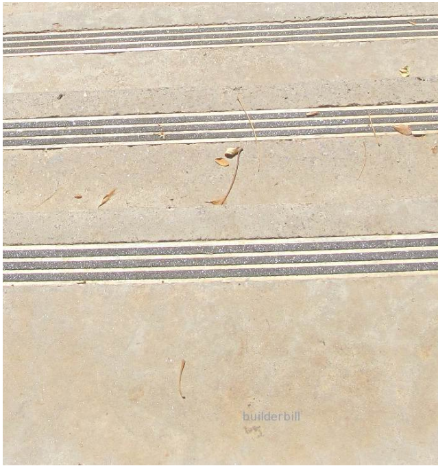
Img 6.1.1: Concrete Nosings
