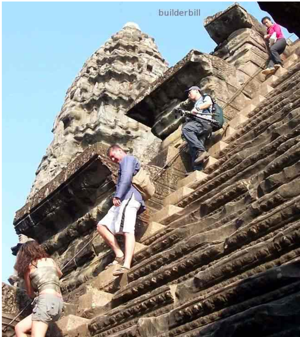
Img 2.0.3: Stairs over the critical angle
