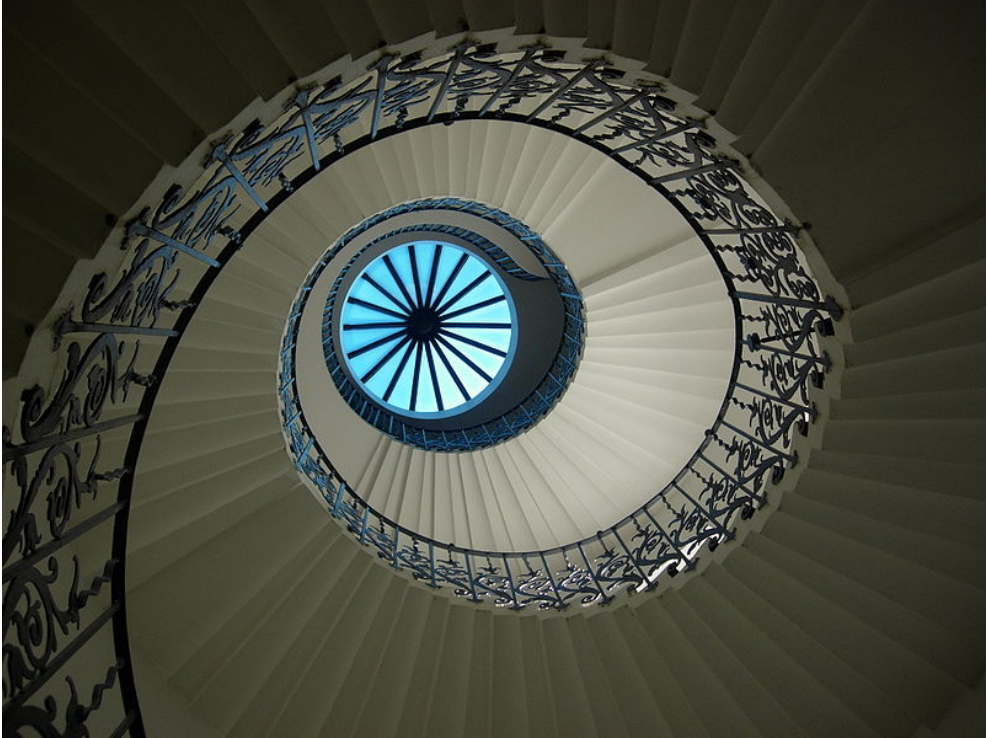
Img 2.0.8: A Cantilever Stone Stair Circa 1670
