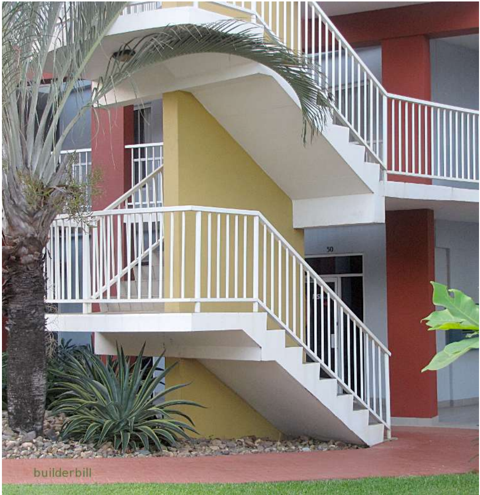
Img 9.0.2: Concrete Cantilever
