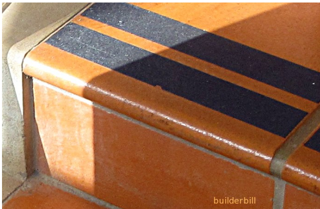
Img 6.1.1: A ceramic bullnose tread
