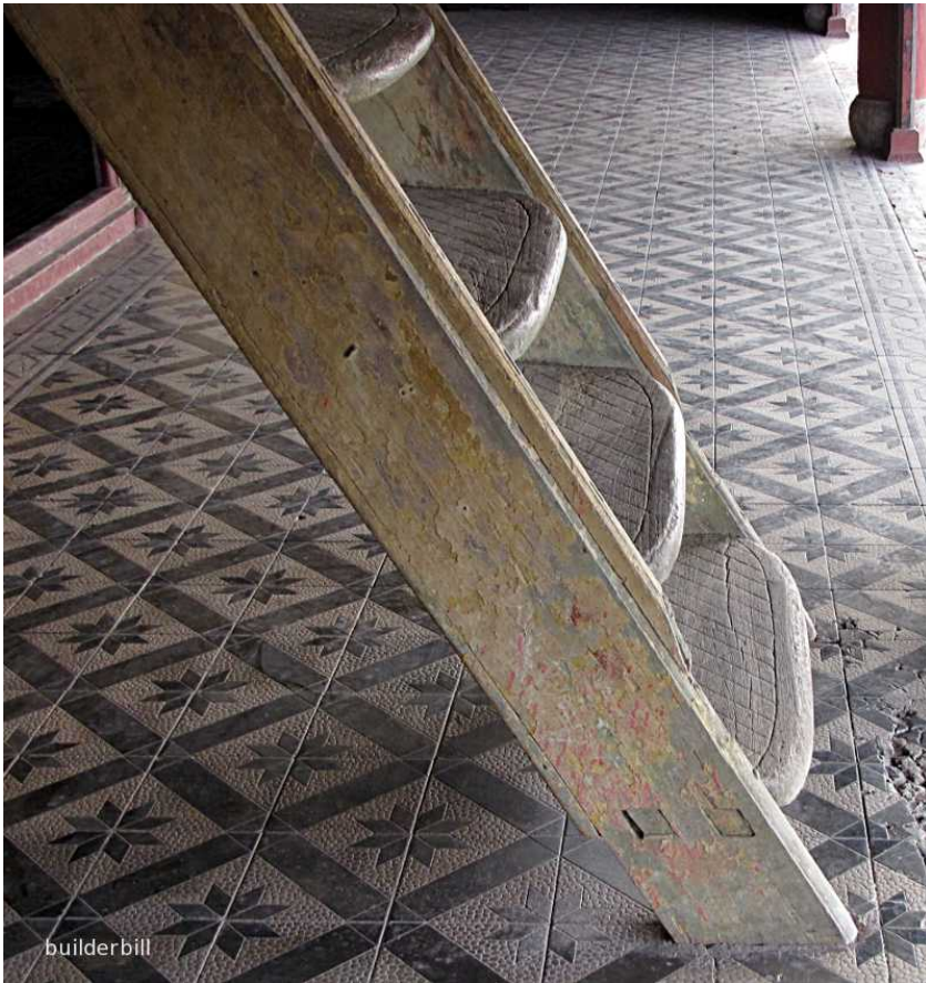
Img 2.0.2: A fixed ladder stair, circa around 1820
