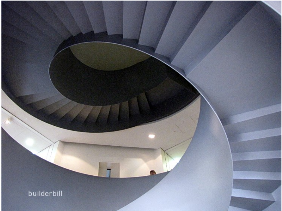
Img 2.0.7: An All Steel Helical Stair from Underneath
