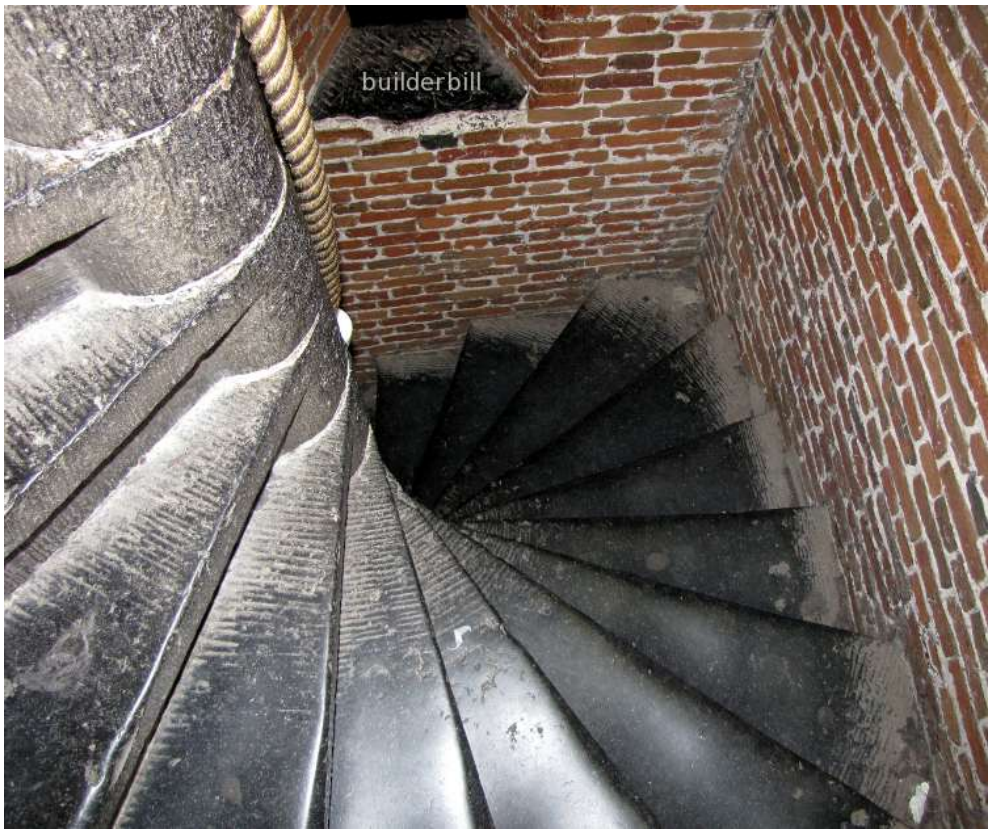
Img 2.0.6: Old Spiral Staircase
