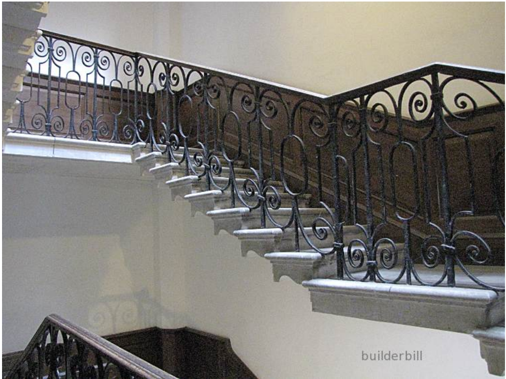
Img 9.0.3: Open Stair
