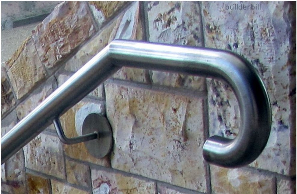
Img 7.0.2: Wall Rail
