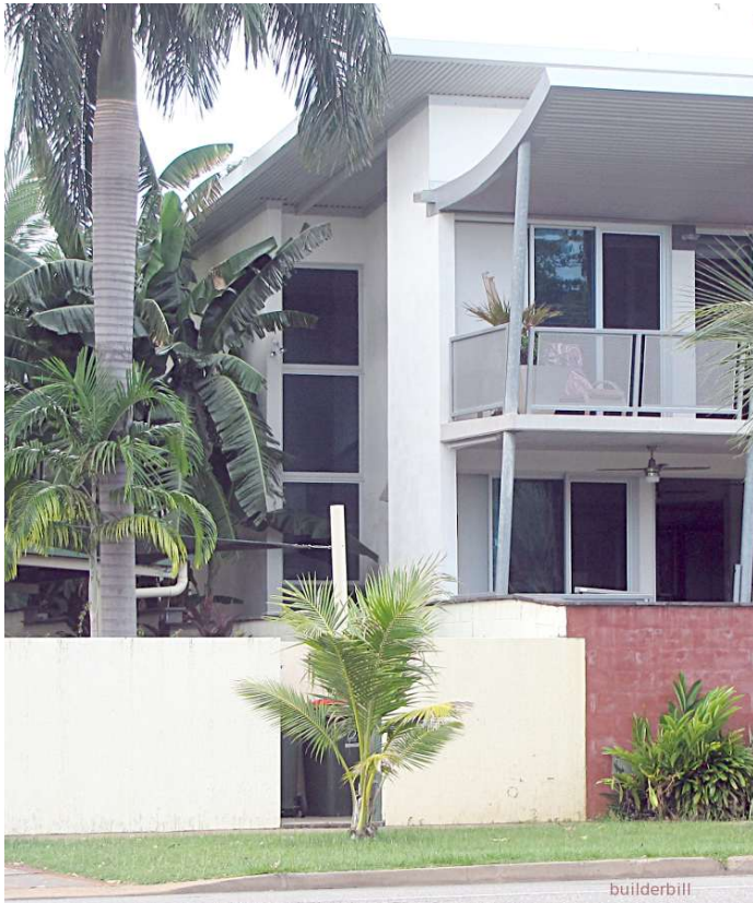
Img 11.2.1: Stairwell windows
