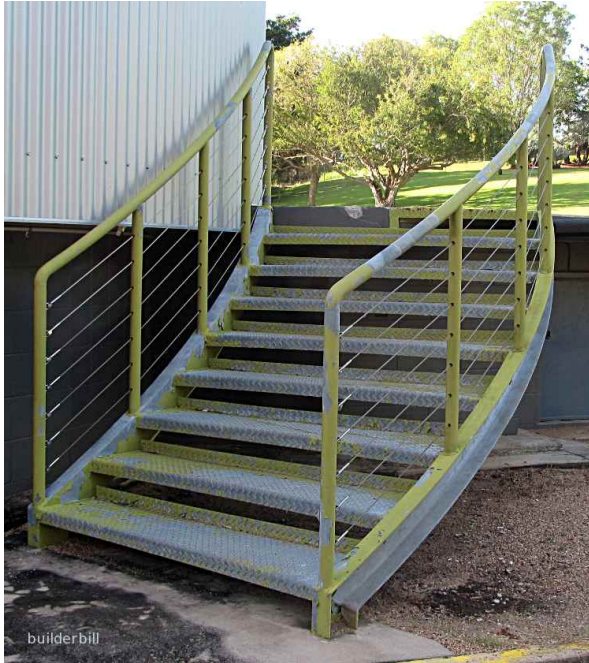
Img 5.5.1: Helical stair, tapered treads
