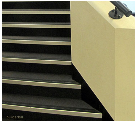
Img 6.1.2: Carpeted treads with metal nosings
