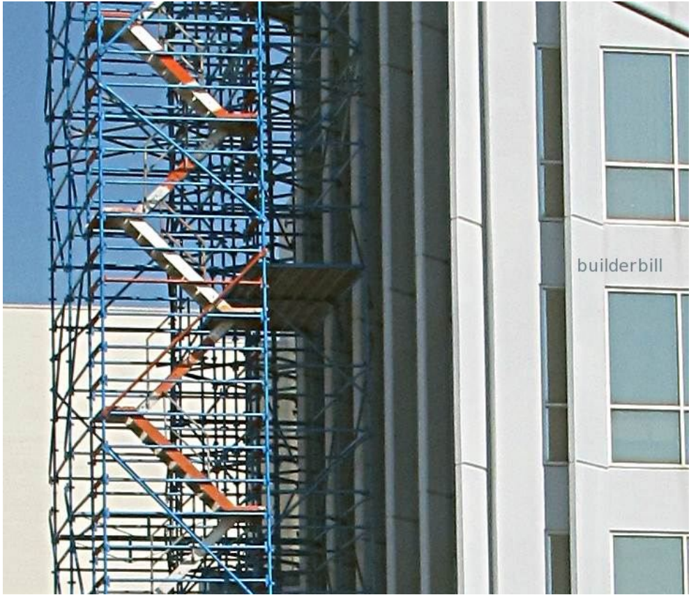
Img 2.0.9: Temporary stair tower
