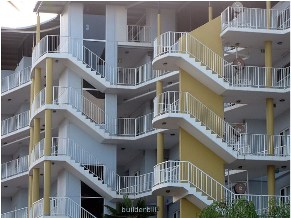
Img 7.1.1: Concrete Stairs and Steel Balustrades
