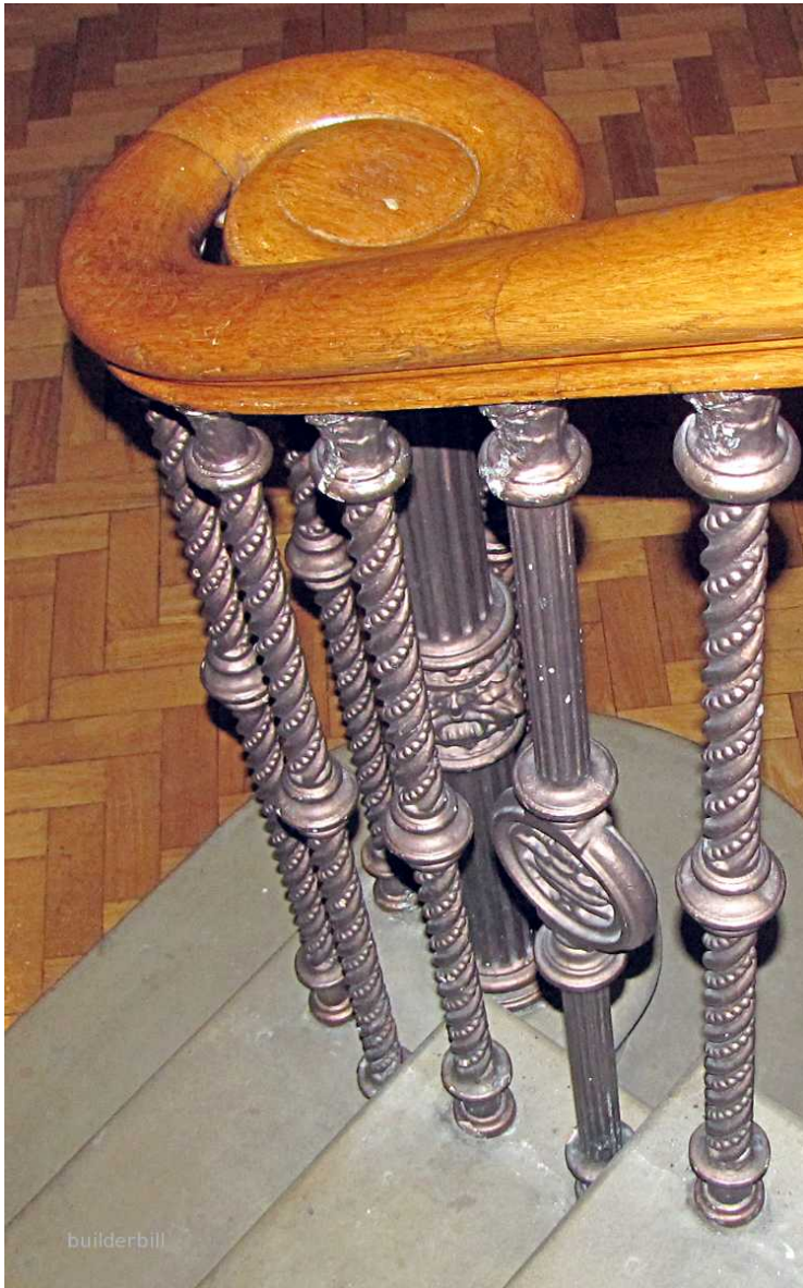
Img 7.0.8: Cast Iron Balusters
