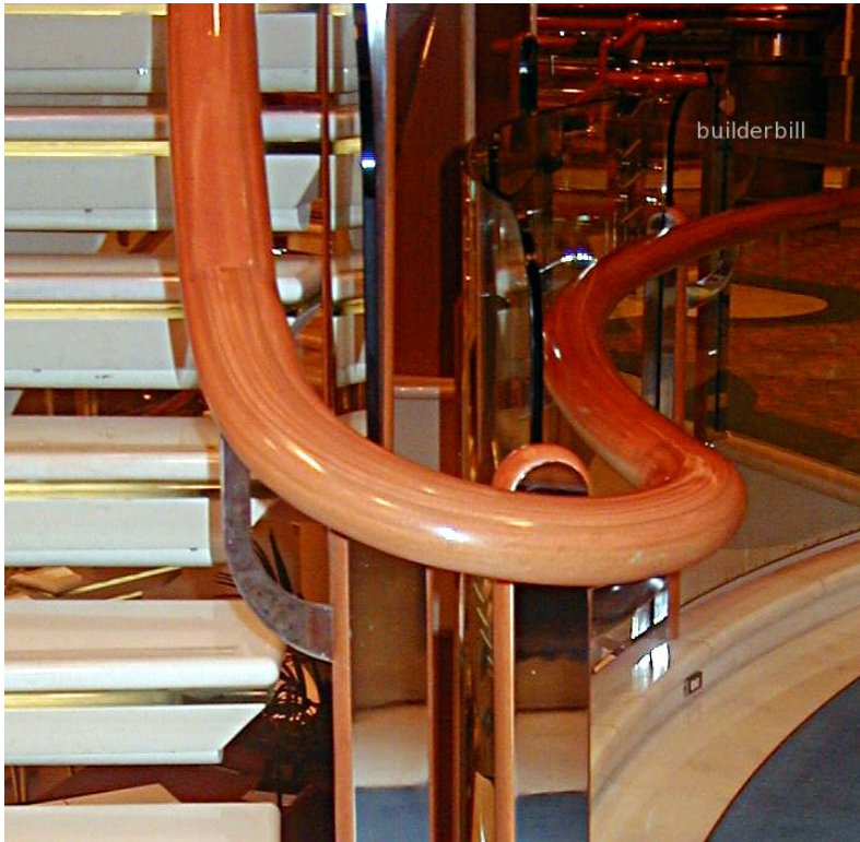
Img 7.1.4: A Modern Continuous Handrail
