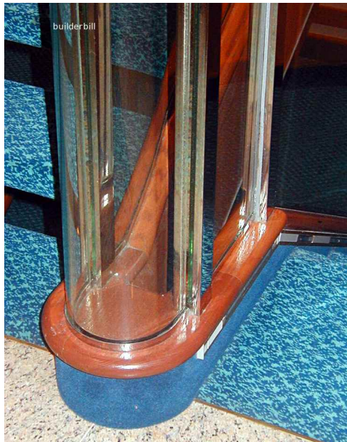
Img 8.1.5: An “L” shaped landing edge
