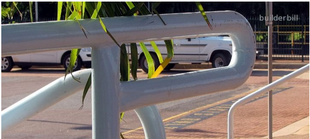
Img 7.0.7: Steel Pipe Rails
